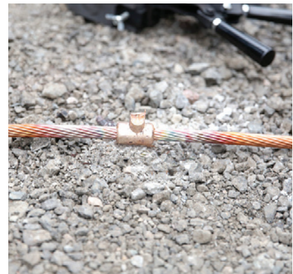
6. Remove weld and clean mold before making next connection.
