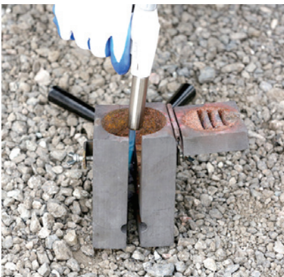
1. Position cleaned conductors in mold after making sure mold is dry, by pre-heating or making a test joint.
